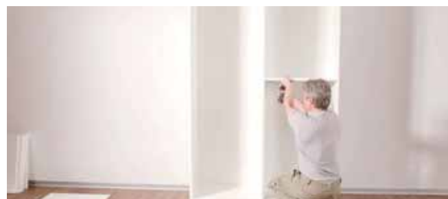
Screw front corner in place with a cordless drill. This makes one-man assembly easy.
