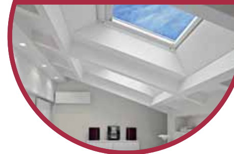
Roof window casing
